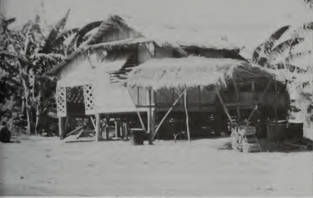
Typical rural Philippine nipa house, constructed of locally available bamboo and nipa-leaf thatching Courtesy Patricia V. Dolan
